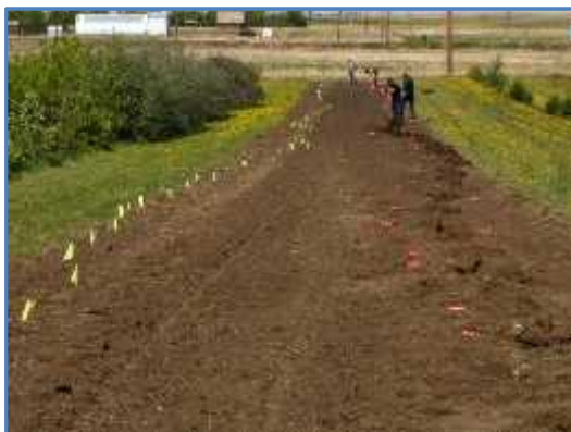
Digging holes to plant the saplings
